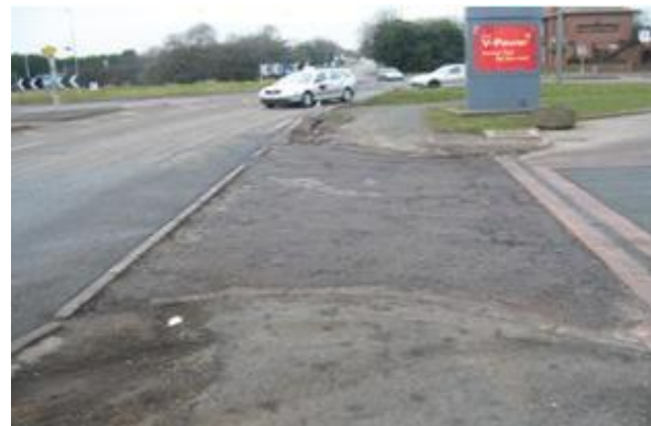
Pothole in other areas >25mm or >150mm diameter
